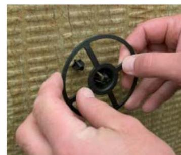
... which is pushed on afterwards as far as the insulation material.
